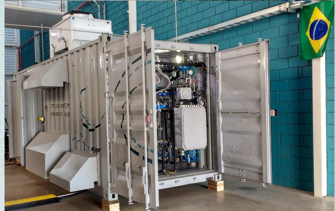
PEM Electrolyser under Comissioning
